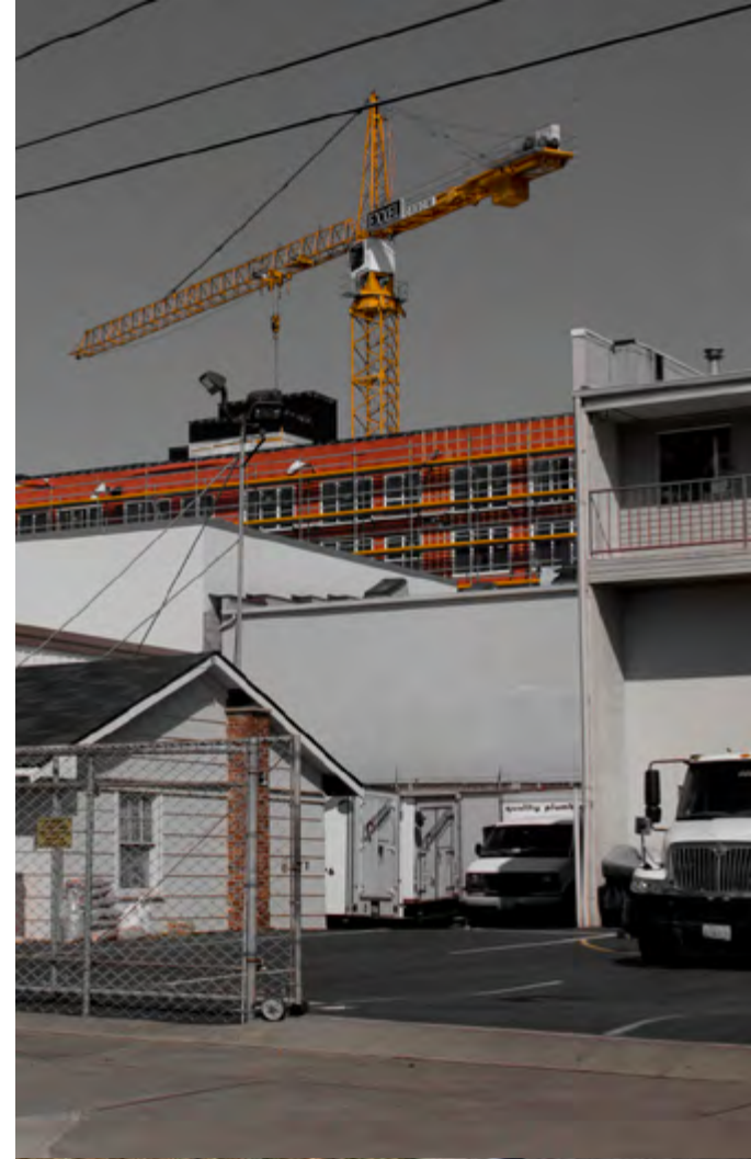
figure 1.03 Construction on the fringe
